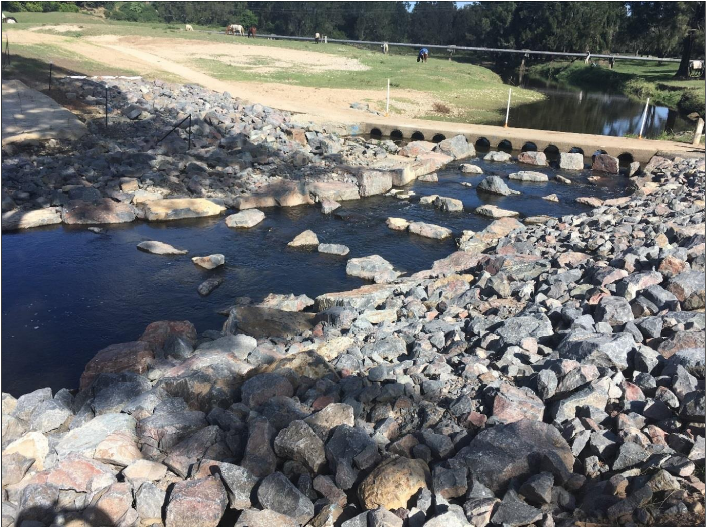
Figure 3. South Pine River fishway at Leitch's Crossing in Brendale, retrofitted to a pedestrian causeway under state development approval in 2017.
