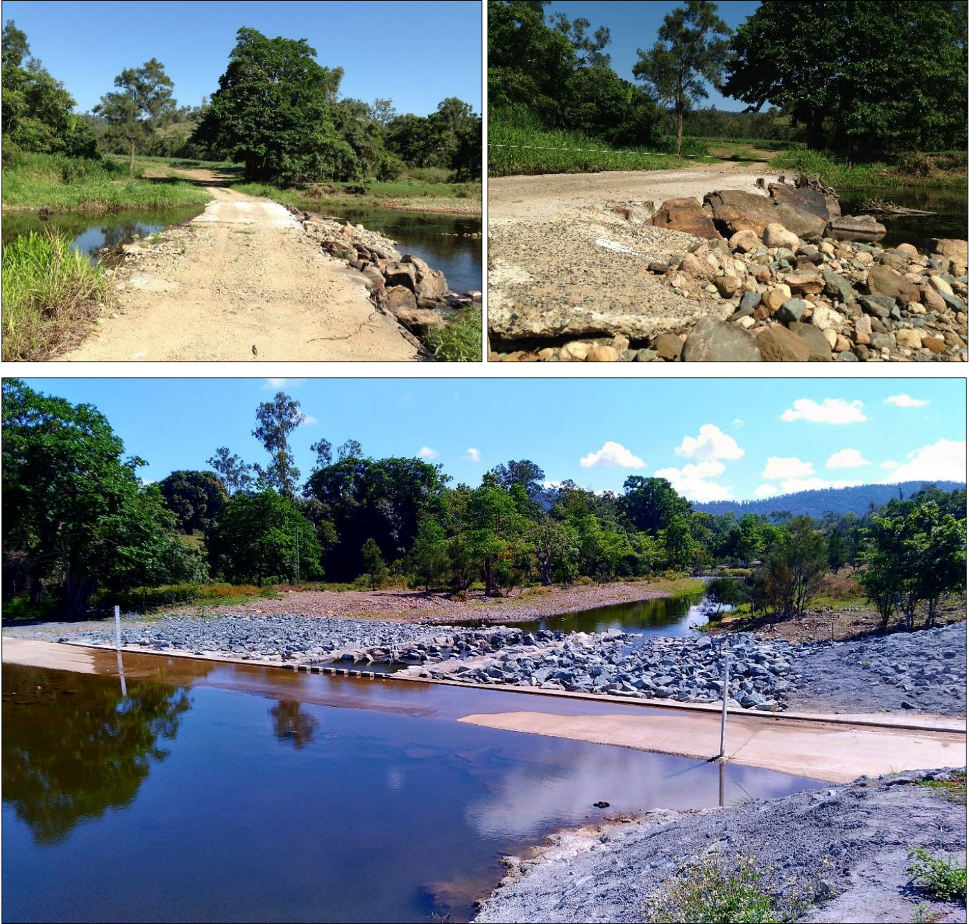
Figure 1. Clews Road causeway was upgraded in 2019 with a concrete flooded causeway. Fish passage provisions incorporated a low flow rock ramp and high flow graded scour protection to the width of the main channel.
