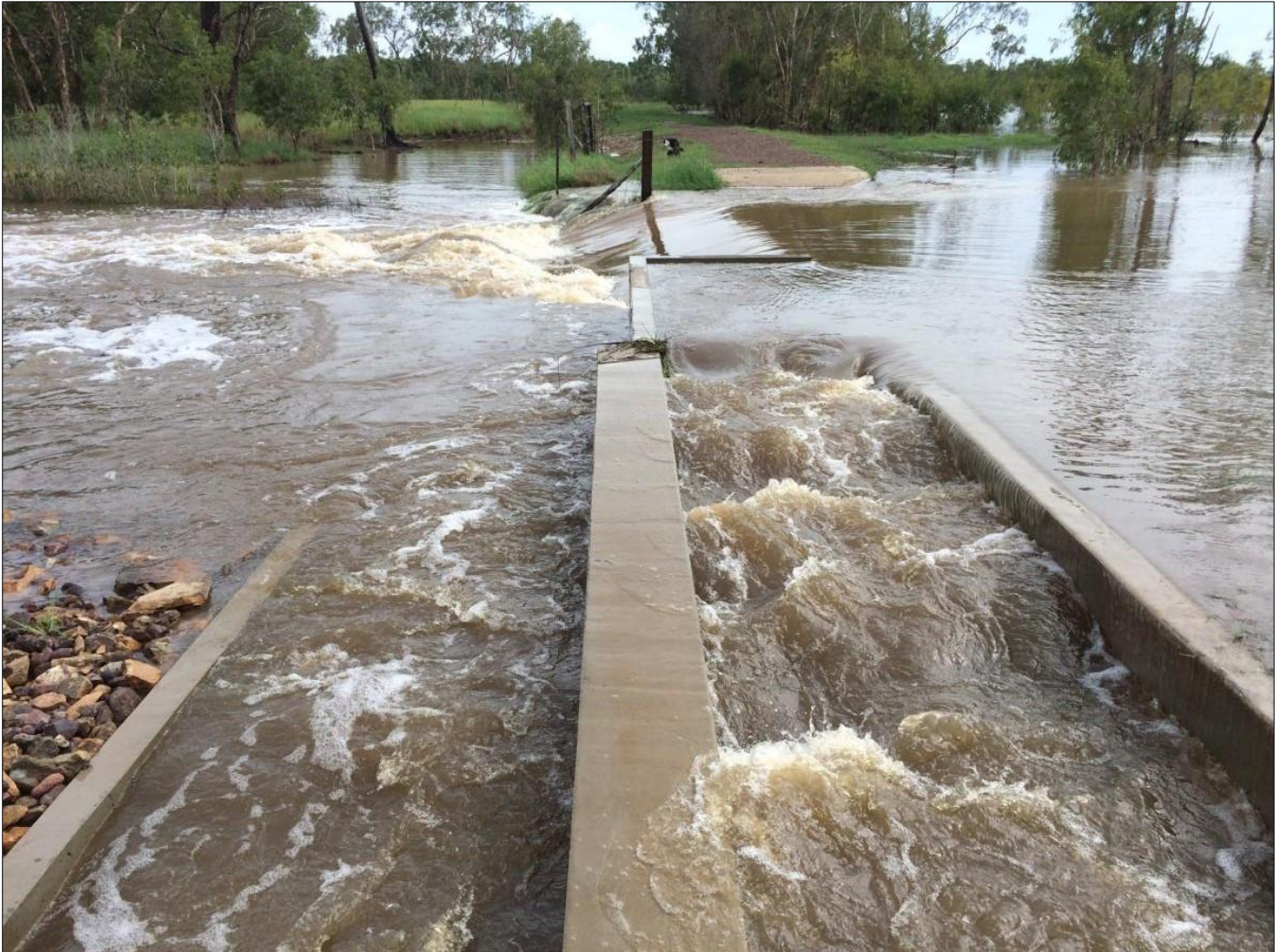
Figure 4. Boundary Creek cone ramp fishway was retrofitted to a ponded pasture spillway to provide connectivity between the estuary and wetland nursery fish habitats upstream.
