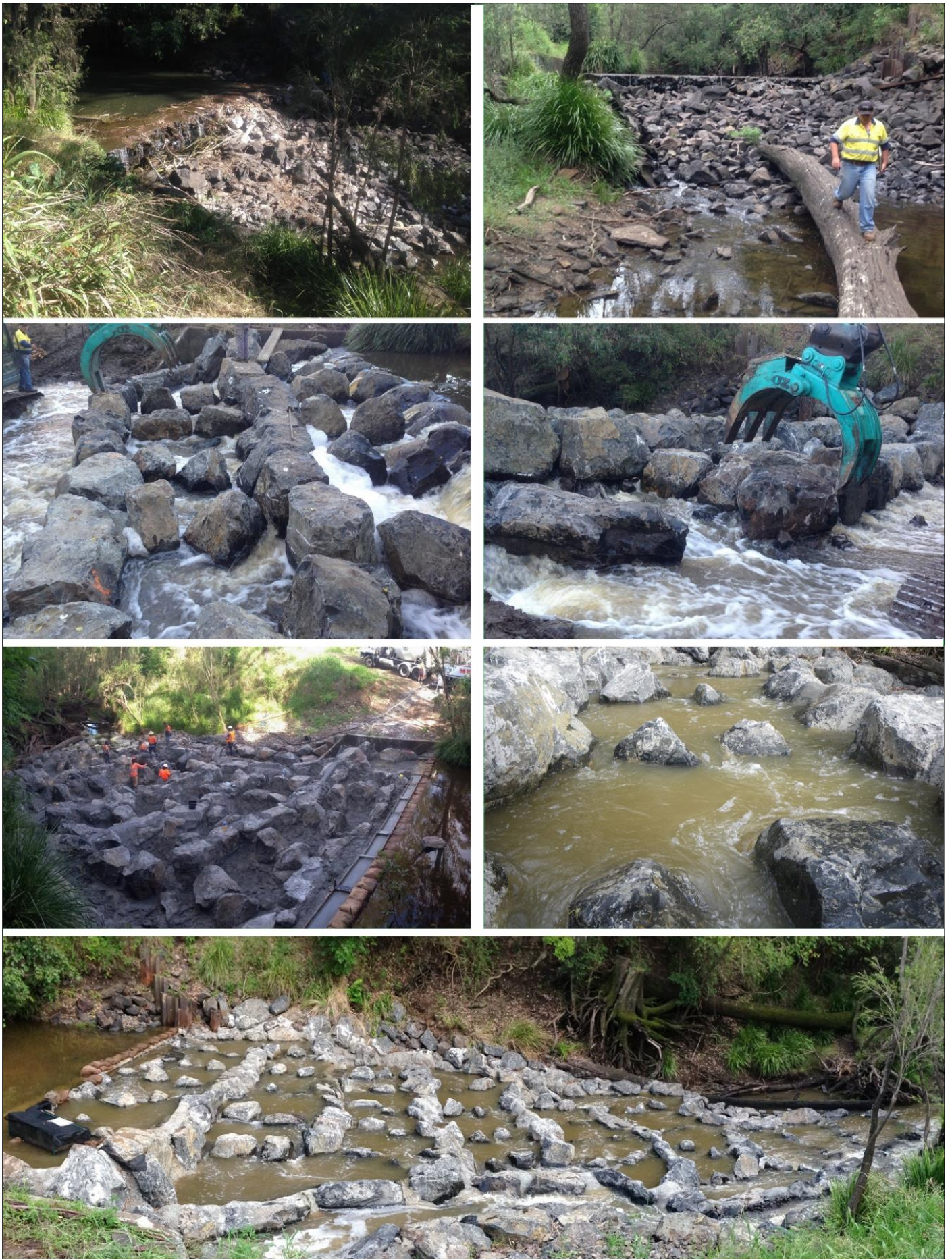
Figure 2. Berry's weir on the Bremer River at Ipswich, A historic weir retrofitted with the longest rock-ramp fishway in Queensland.
