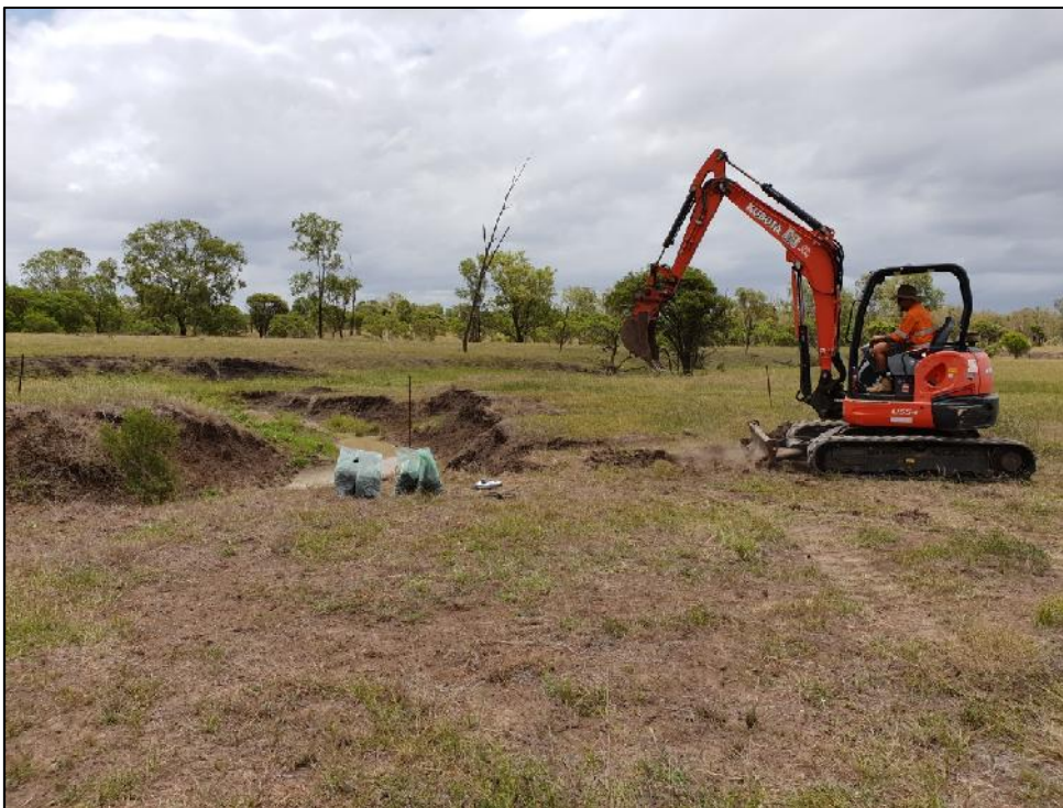
Figure 2: Photo looking approximately North to incised dam wall (left), with excavator backfilling Test Pit 7.
