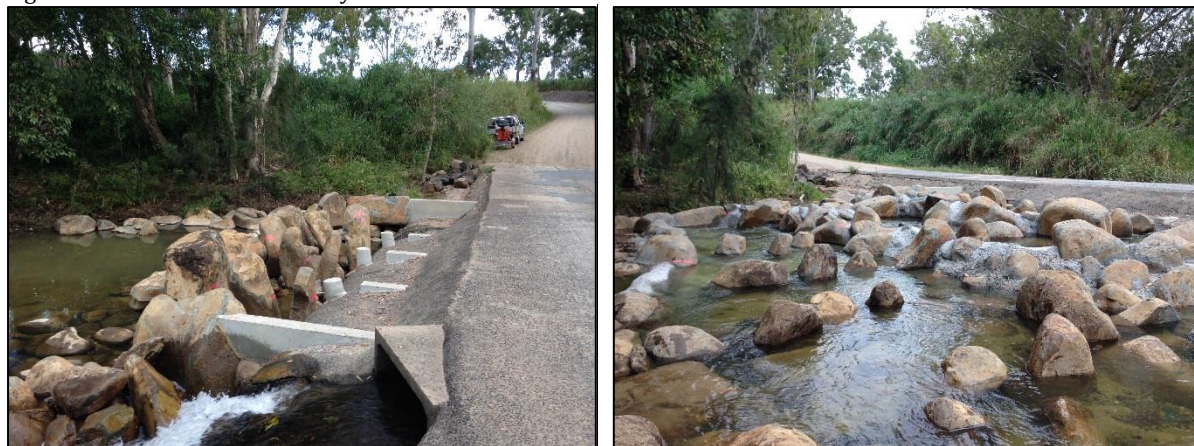
Figure 5. Blackrock Creek fishway during construction (left) and shortly after completion (right).
