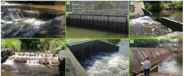
Figure 2. Barrier structures: a) Road causeway & concrete apron (Elimbah Ck), b) tidal floodgates (Behm Ck), c) V-notch stream gauging weir (Warrill Ck), d) Sheet pile and gabion basket weir (Warrill Ck), e) pipe culvert causeway (Albert River) and f) Tidal barrage (Caboolture River).
