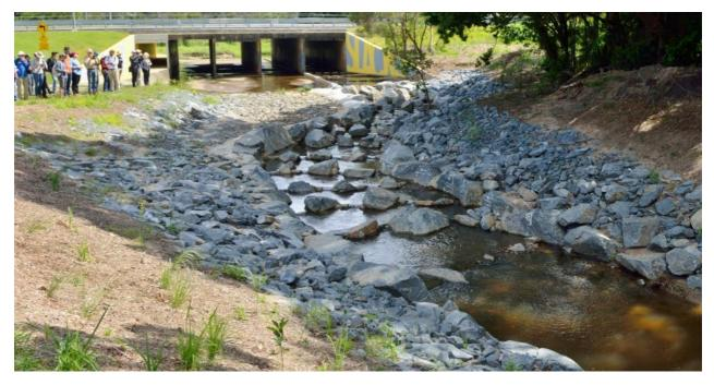
Figure 15. Showing one of the four priority ranked barriers remediated as part of this project; Slacks Creek, (Paradise Road) 17 ridge rock-ramp and horizontal culvert baffle fishway (photo courtesy of Leo Lee).
