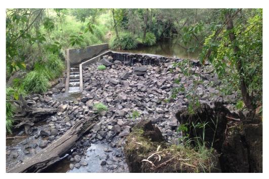
Figure 23. Berrys Weir fish barrier before remediation works, with relict north- American style fish ladder visible down left side of weir
