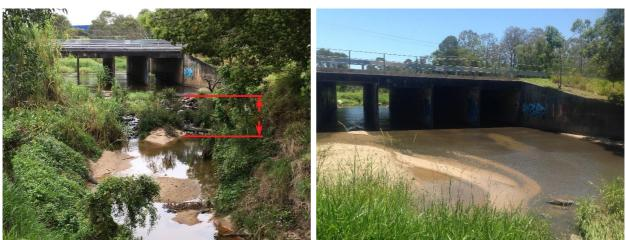
Figure 20. Left; showing the 1.3 m surface drop barrier off the downstream face of the culvert apron. Right; showing stream flow spread out across all four box culverts creating a shallow water surface barrier along the entire 50 m length of the structure. During stream flow events the culverts also created a flow velocity barrier.
