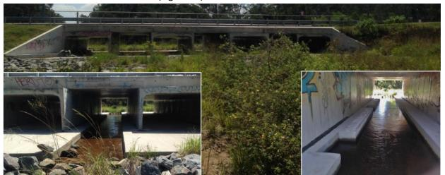
Figure 19. Culvert crossing conforming to Accepted Development requirements. Note: Low flow channel and wall roughening.
