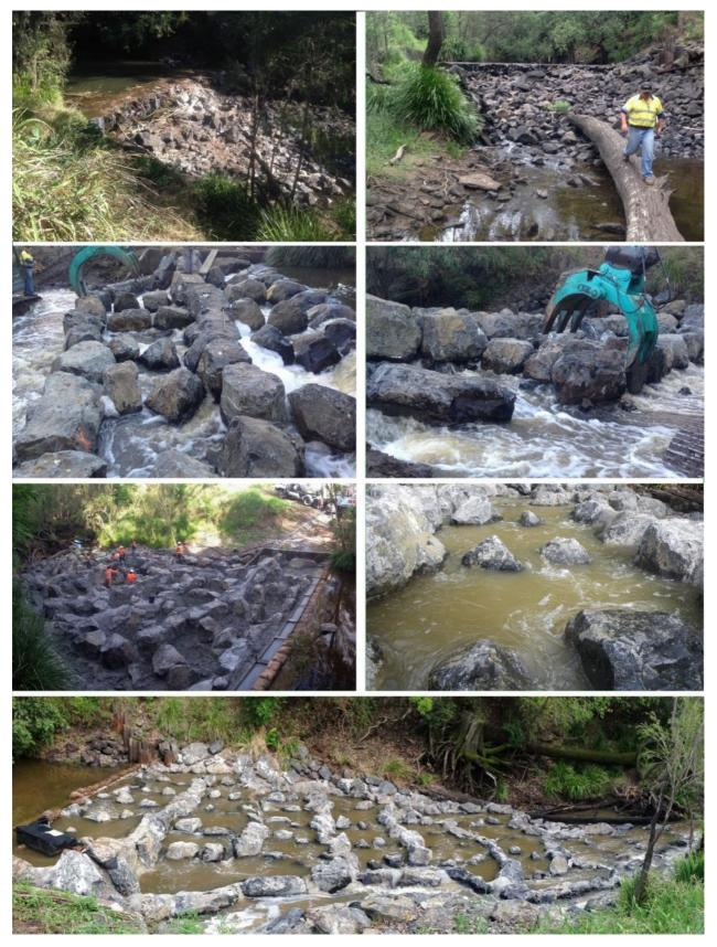
Figure 24. Berrys Weir fishway construction images
