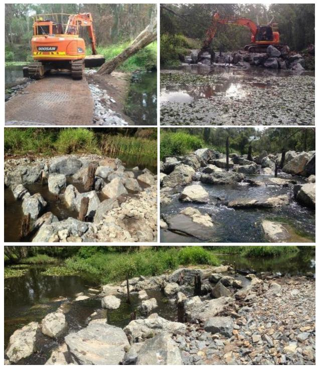
Figure 30. Showing construction images of Hilliards Creek fishway
